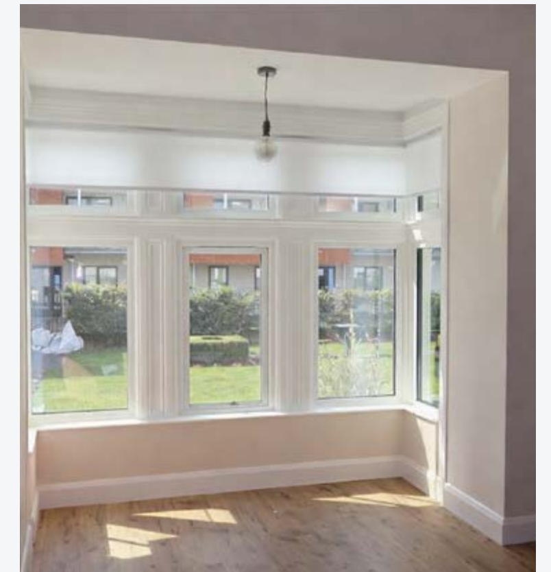
Post upgrade works - triple glazed windows
