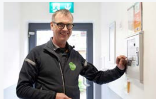
I-RES Maintenance Technician John O'Sullivan carrying out safety checks at the School Yard, Dublin 1
