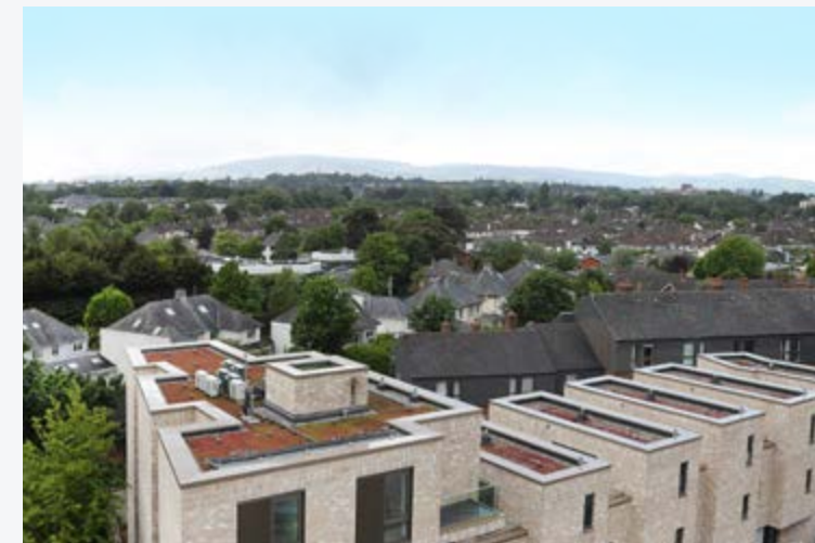
Green roofs at Tara View, Dublin 4
